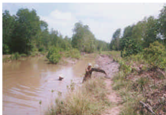
Sediment removal in mangrove-aquaculture farm system
